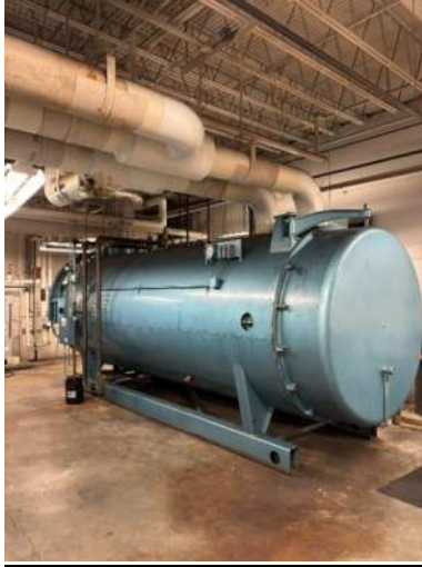
Figure 1 : Existing Oil-Fired Boiler
