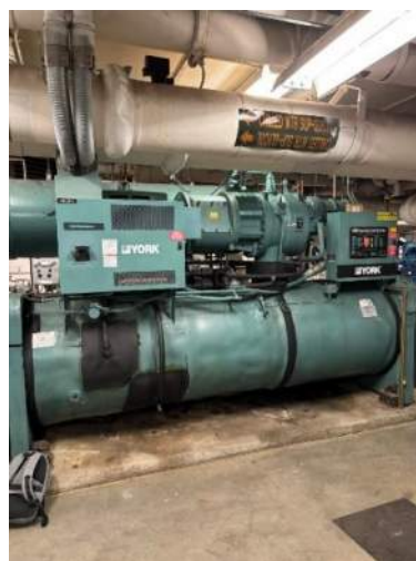
Figure 4: Existing 350-Ton Chiller
