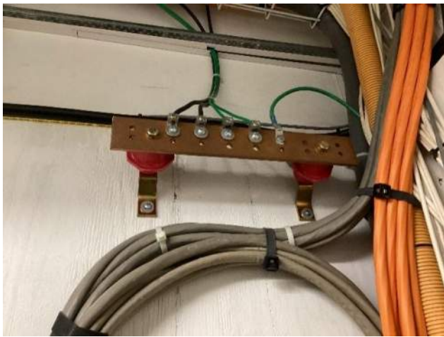
1 Existing bonding busbar in a TR, bonding is not present in all TR's.
