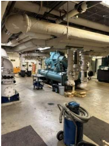
Figure 3 : Existing 525-Ton Chiller
