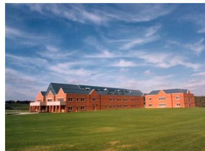
The Great Hall and Classroom Building C in 1990.
