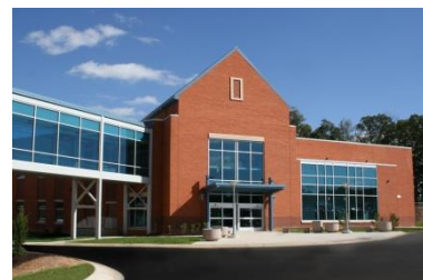
Classroom Bldg. 4 opened in winter 2010.
